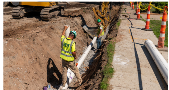
Placing of the perforated PVC pipes into the trenches.
